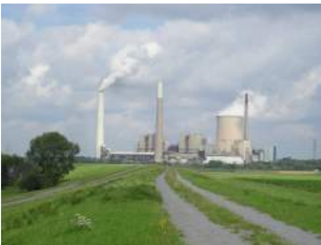
Another Identical Power Station
